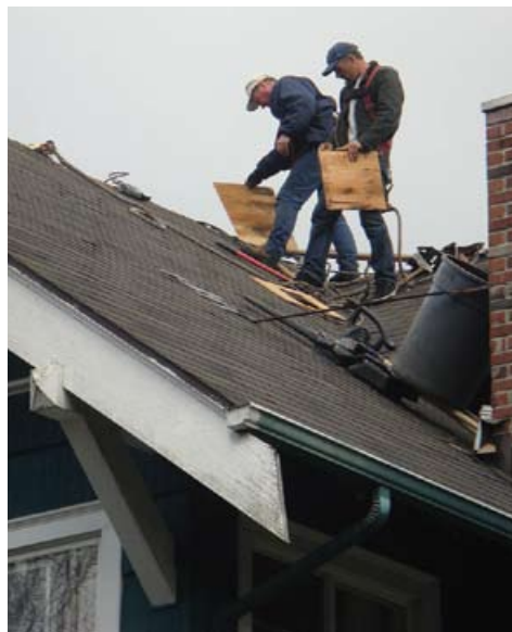
Group Home getting new roof!
